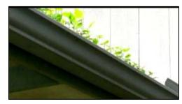
**Cover Up:** Place mesh over gutter to prevent future debris from accumulating.
